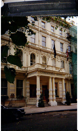
...to Square, 1998, the two windows left on the 2nd floor above the www.oreta-ransom.com ...
